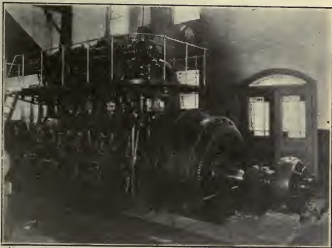
INTERIOR OF FREEPORT, L. I., POWER-PLANT, SHOWING DIESEL ENGINE INSTALLATION
